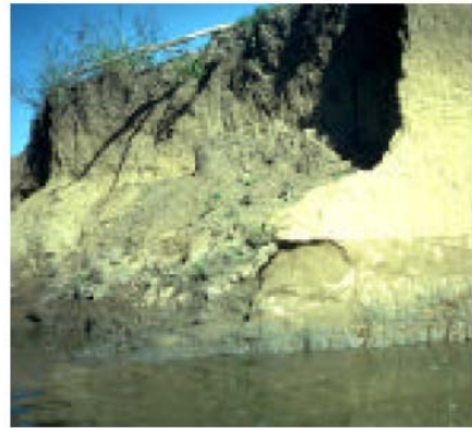
Severe bank erosion.
