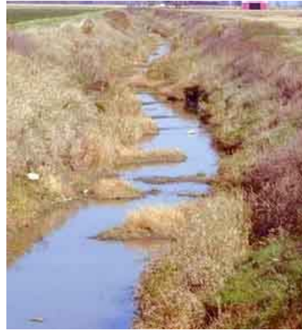
A channelized stream channel starting to revert towards more natural channel features.
